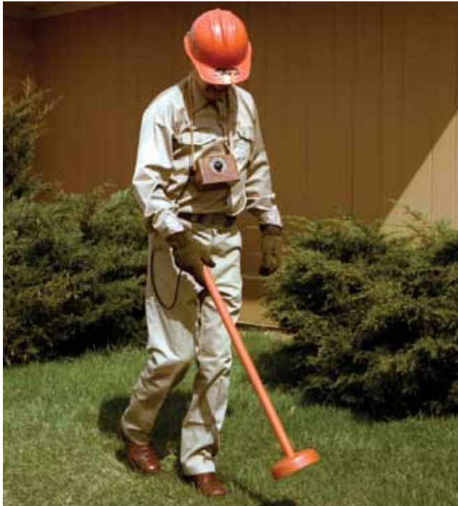
Locating the buried cable (Cat. No. T4030572)
